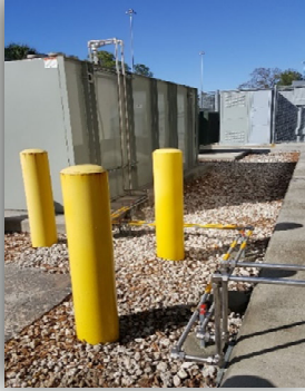
CNG Compliance Repairs, HART's 21st
