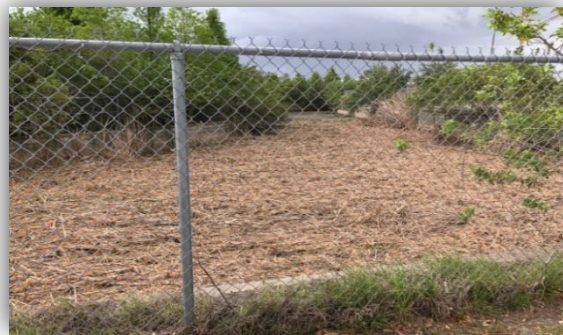
Ruskin Park-N-Ride Stormwater Pond Clearing
