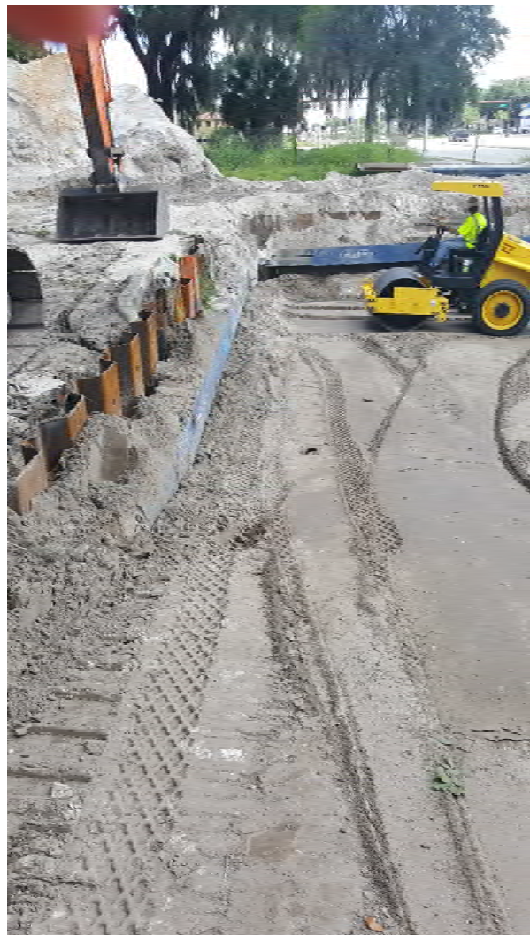
Source Removal, Moore Haven, FL
